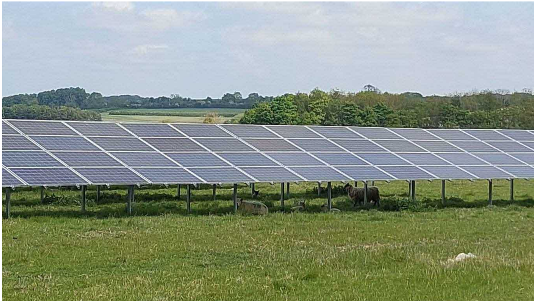
Plate 1: Typical Solar Panel Arrangement –Landscape Formation
